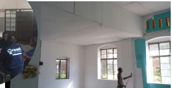
Planning & renovation process for the new look Pugu library
