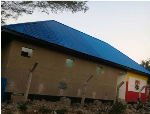
Construction at an advanced stage
