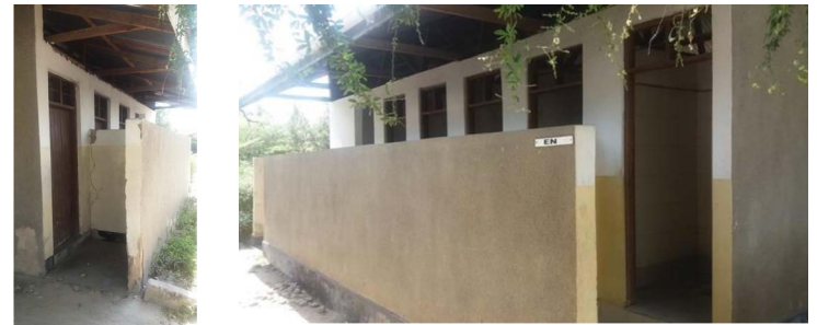
Latrine system used by the school before intervention
